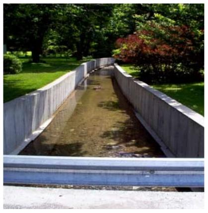
Looking upstream from Quinton Court at the channelization of the stream. This structure concentrates discharge velocities in the stream, which impacts the stream channel downstream.
