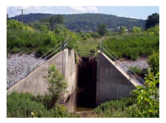
View of the diversion structure outlet. Here diverted water outlets into the Rugg Brook.
