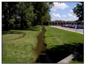
Straightened channels and lack of vegetated buffer reduces ability to filter pollutants from parking lots and contributes to flooding.
