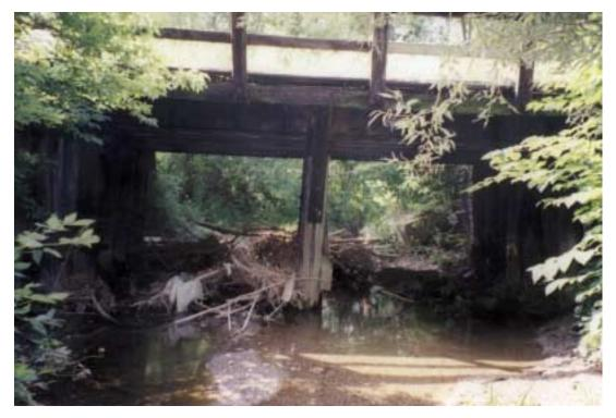
View looking upstream of a railroad bridge crossing the Stevens Brook. Note the debris accumulating in the stream due to the support pier.
