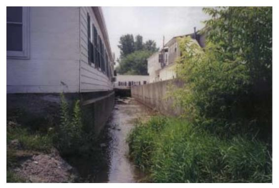
View looking upstream of the Lake Street crossing. The stream has been confined to this narrow channel because of the encroachment.
