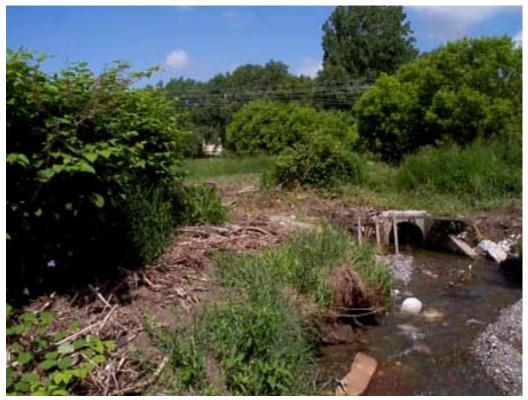
Inlet of the control culvert on Stevens Brook. When discharges exceed capacity of this culvert, water is diverted into the diversion structure and conveyed to the Rugg Brook outlet shown in the next photo.
