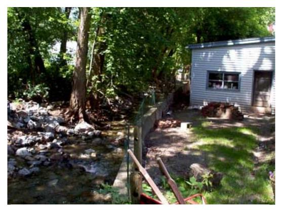
Another view of the floodwall along Lower Weldon Street. It is at this location that flooding frequently occurs. This area is a natural floodplain and the wall is marginally effective in containing the stream during significant discharges the stream overtops the wall and floods the property shown at the right.
