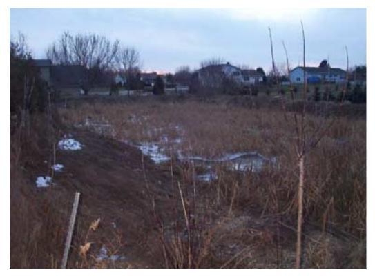
A view of an unmaintained detention basin. Unmaintained detention basins do not operate as intended and often result in localized flooding and adverse impacts on the receiving stream.
