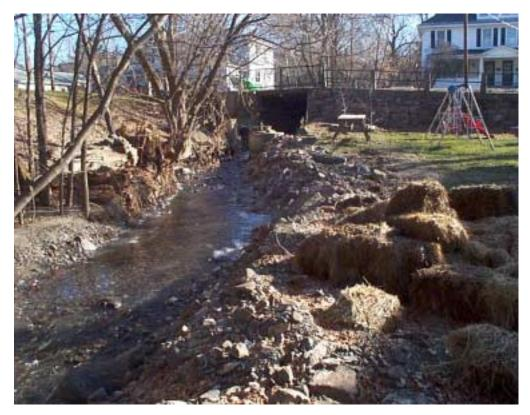
Upstream view of the Barlow St. culvert. This area is frequently inundated at which time sediment is deposited on the residential property. Note the absence of any riparian vegetation. Also note the berm adjacent to the stream, which was constructed by the property owner from sediment deposited by the stream.
