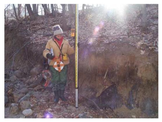
View of left bank of the Stevens Brook along the reach between Lincoln Ave. and Main St. Note the significant streambank erosion caused by excessive stormwater discharge.
